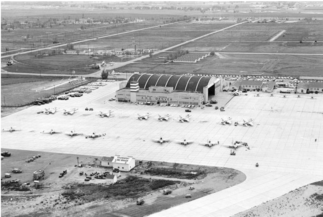
Figure 5. Naval Reserve Hangar, Buckley Field, ca. 1950. United States Air Force photograph from author's collection.
