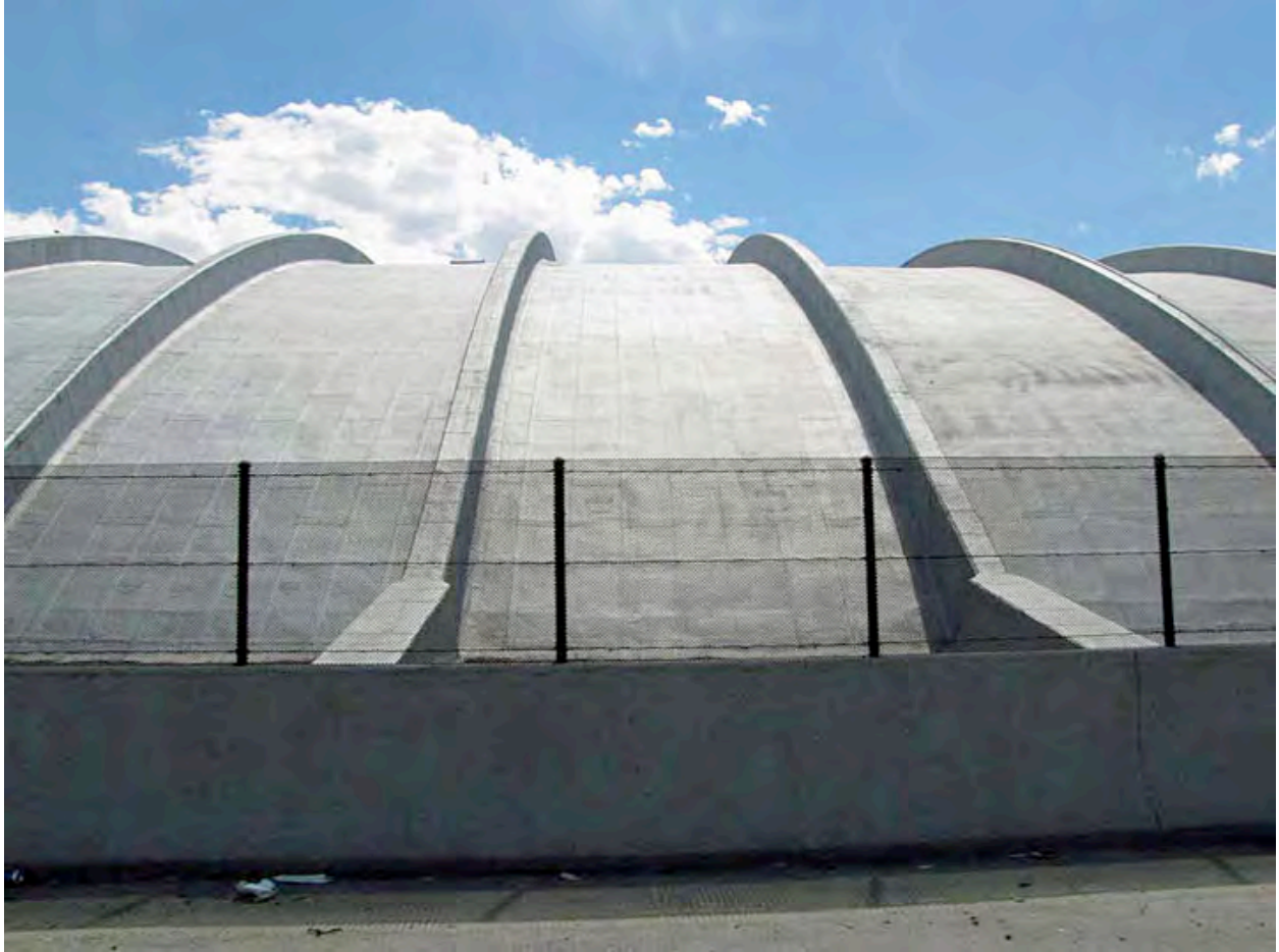
Figure 12. Denver Coliseum. Arch roof surface and supporting ribs as seen from Interstate 70, view to the south from eastbound lane. Photograph © Scott D. Murdock, 2010.
