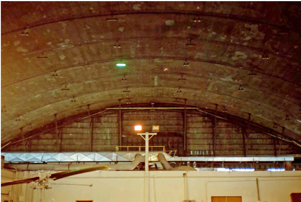
Figure 9. Ellsworth Air Force Base. Thin-shell concrete hangar, interior. Photograph © Scott D. Murdock, 2001.
