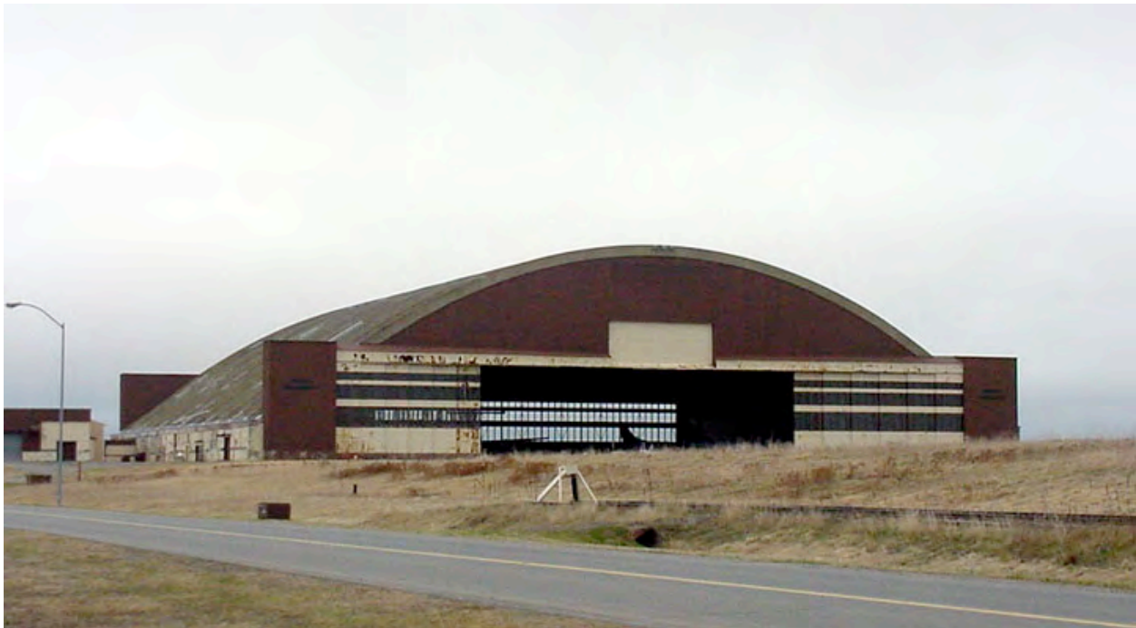
Figure 7. Loring Air Force Base. Thin-shell concrete hangar, exterior. Photograph © Scott D. Murdock, 2004.
