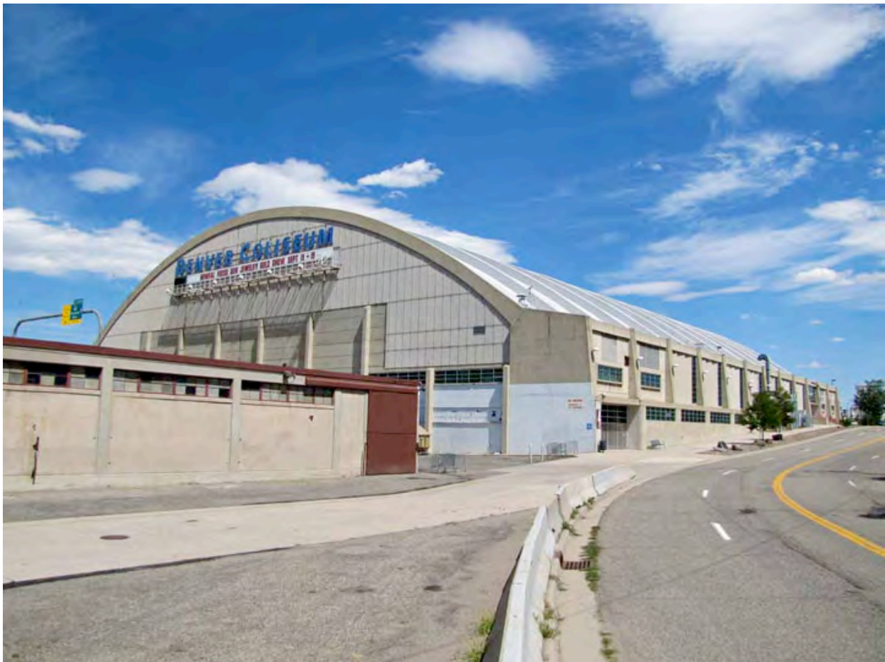
Figure 11. Denver Coliseum (right) and “barn” (left). Connecting “annex” not visible. Photograph © Scott D. Murdock, 2010.
