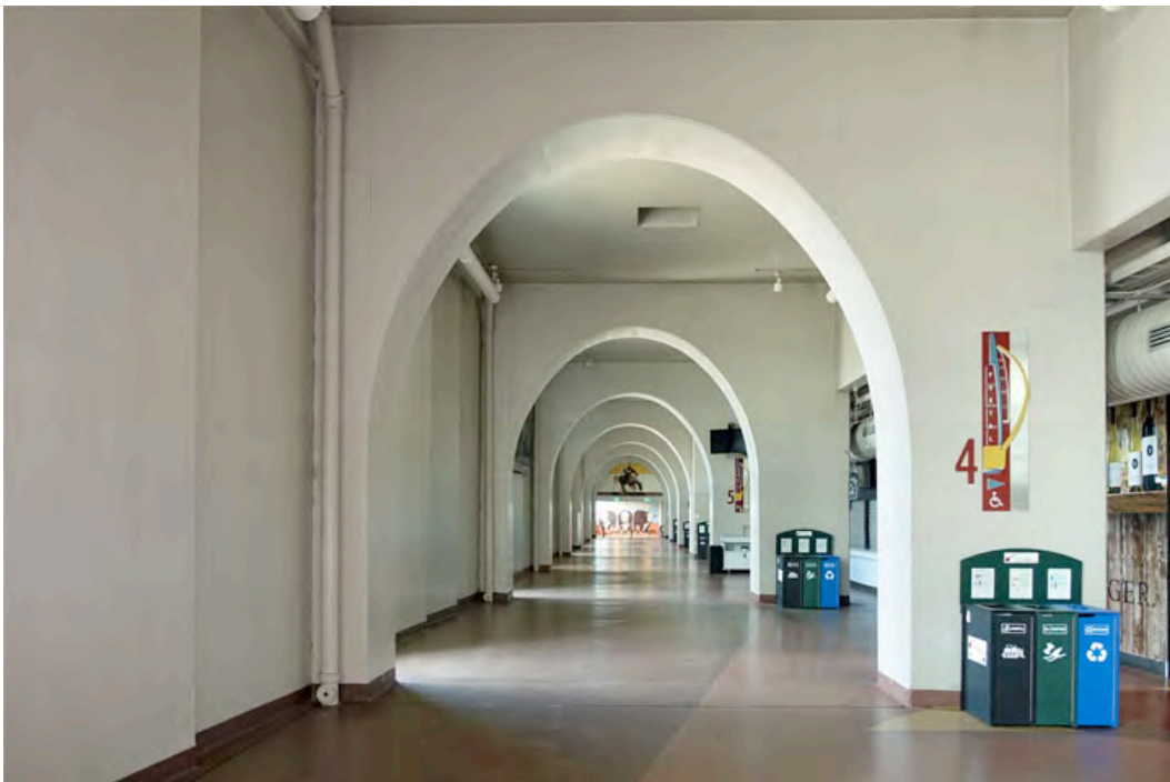
Figure 14. Denver Coliseum. South promenade under concrete arch buttresses. Photograph © Scott D. Murdock, 2016.
