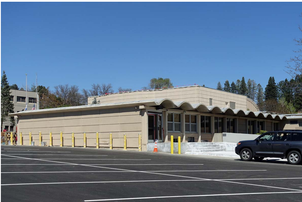
Figure 8. Jewish Community Center, Denver. Multiple buildings with undulating barrel shells. Photograph © Scott D. Murdock, 2017.
