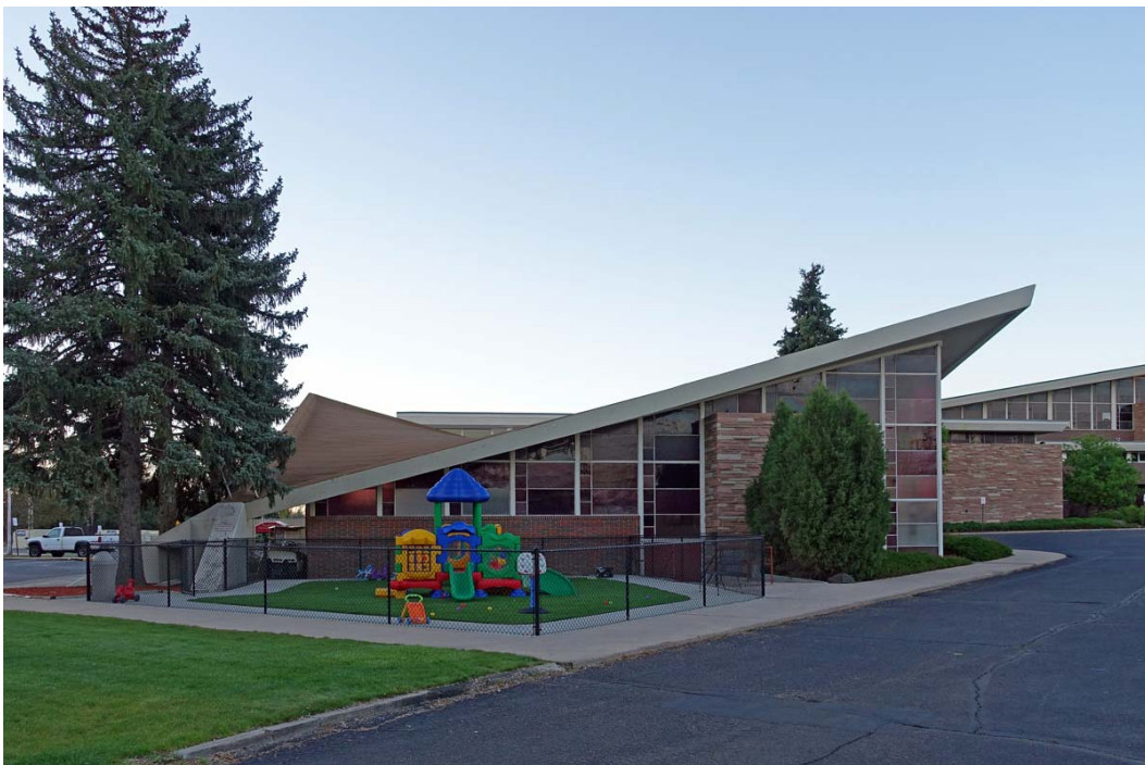
Figure 10. Calvary Temple, Denver. Single hyperbolic paraboloid. Photograph © Scott D. Murdock, 2017.
