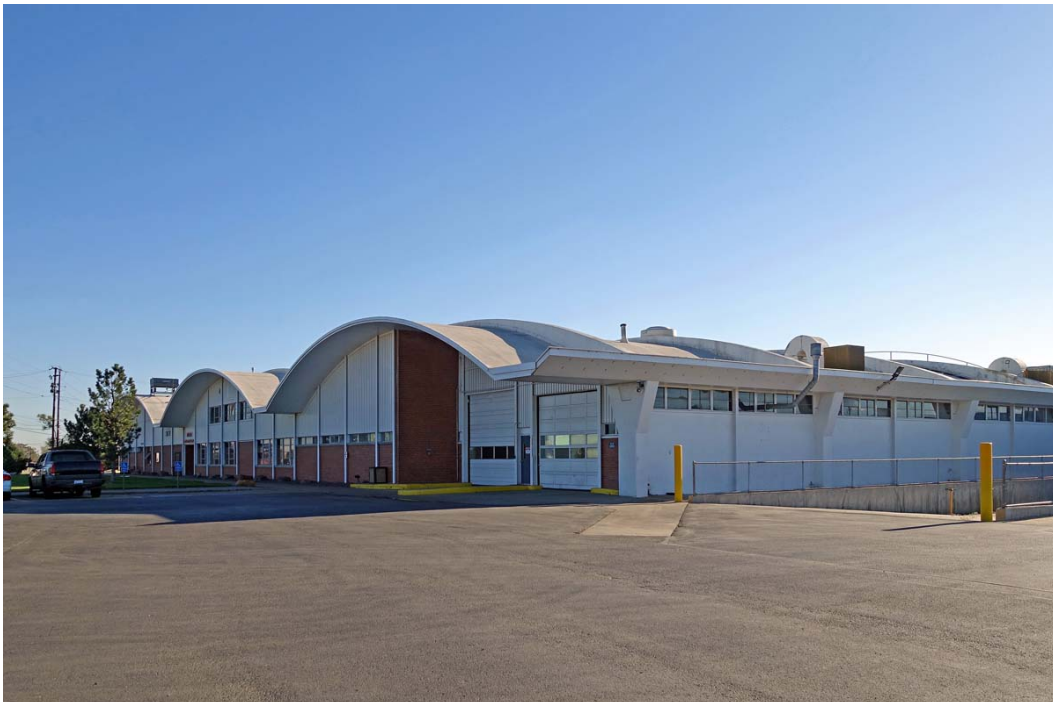
Figure 6. Rainbo Bakery, Commerce City. Three catenary barrel shells. Photograph © Scott D. Murdock, 2017.
