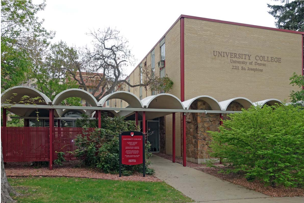
Figure 9. University College, Denver. Multiple barrel shells. Photograph © Scott D. Murdock, 2017.
