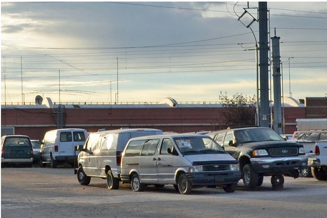
Figure 4. Western Electric Warehouse, Denver. Multiple barrel shells. Photograph © Scott D. Murdock, 2016.
