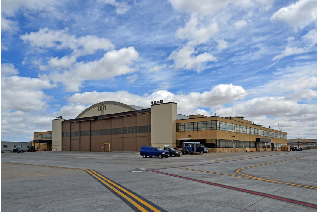
Figure 1. Naval Reserve Hangar, Buckley Air Force Base. Single barrel shell. Photograph © Scott D. Murdock, 2017.
