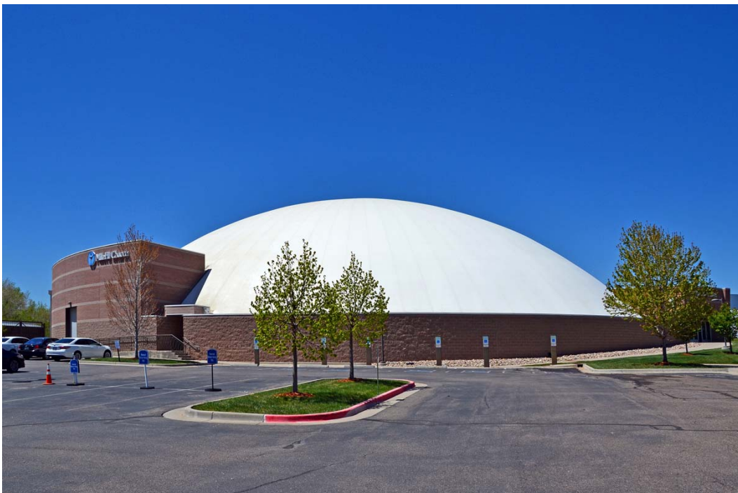
Figure 14. Mile Hi Church, Lakewood. Large, air-inflated dome. Photograph © Scott D. Murdock, 2017.
