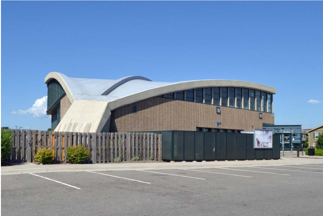
Figure 7. Ideal Cement Company Hangar, Denver. Single barrel shell, diamond shaped. Photograph © Scott D. Murdock, 2016.
