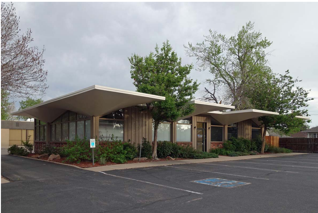
Figure 12. Office Building, Littleton. Eight inverted umbrella hyperbolic paraboloids. Photograph © Scott D. Murdock, 2017.
