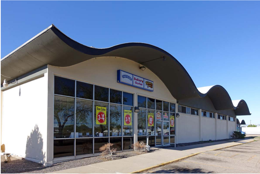
Figure 5. Continental Bakery, Denver. Multiple undulating barrel shells. Photograph © Scott D. Murdock, 2017.
