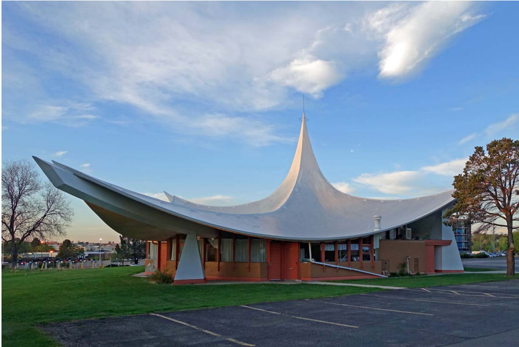
Figure 11. St. Stephens Lutheran Church, Northglenn. Four hyperbolic paraboloids. Photograph © Scott D. Murdock, 2017.
