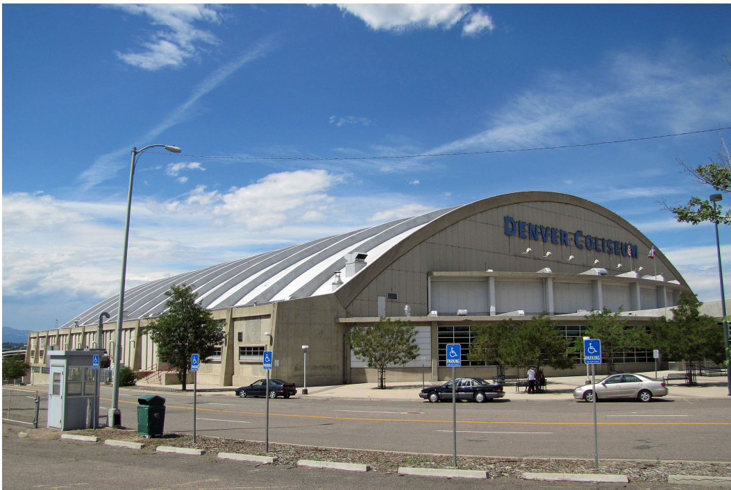
Figure 2. Denver Coliseum, Denver. Single barrel shell. Photograph © Scott D. Murdock, 2016.
