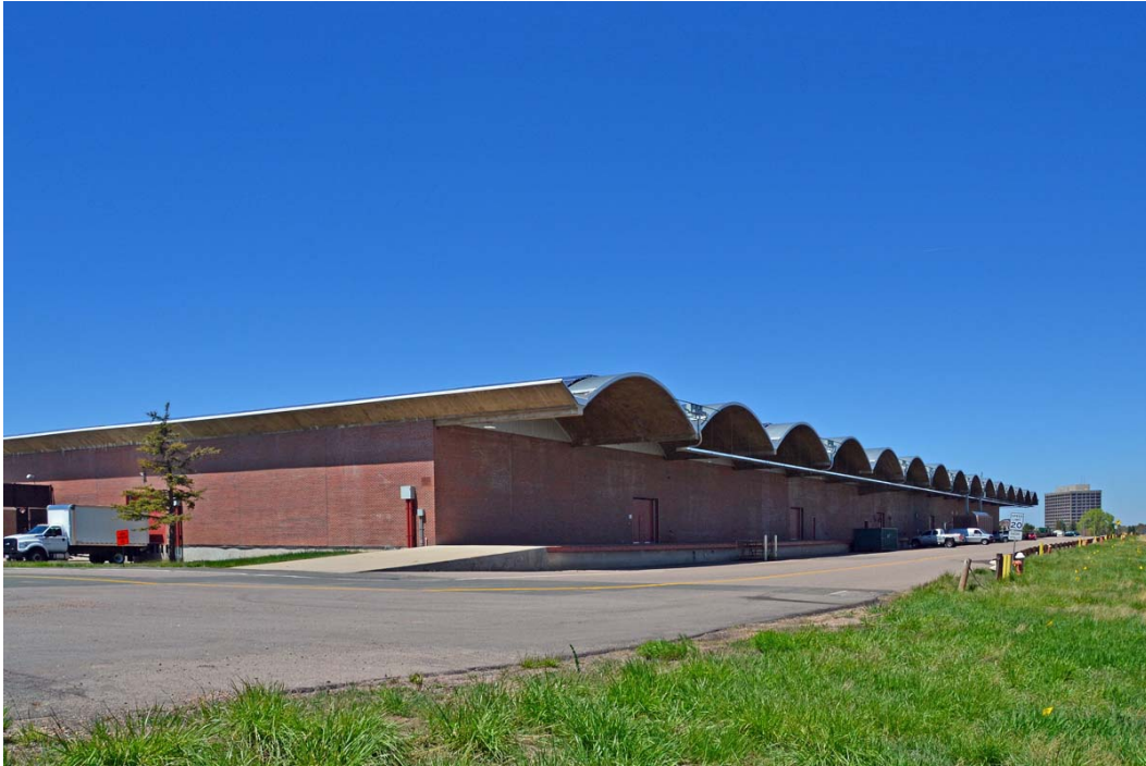
Figure 3. Denver Federal Center Warehouse, Lakewood. Multiple barrel shells. Photograph © Scott D. Murdock, 2017.
