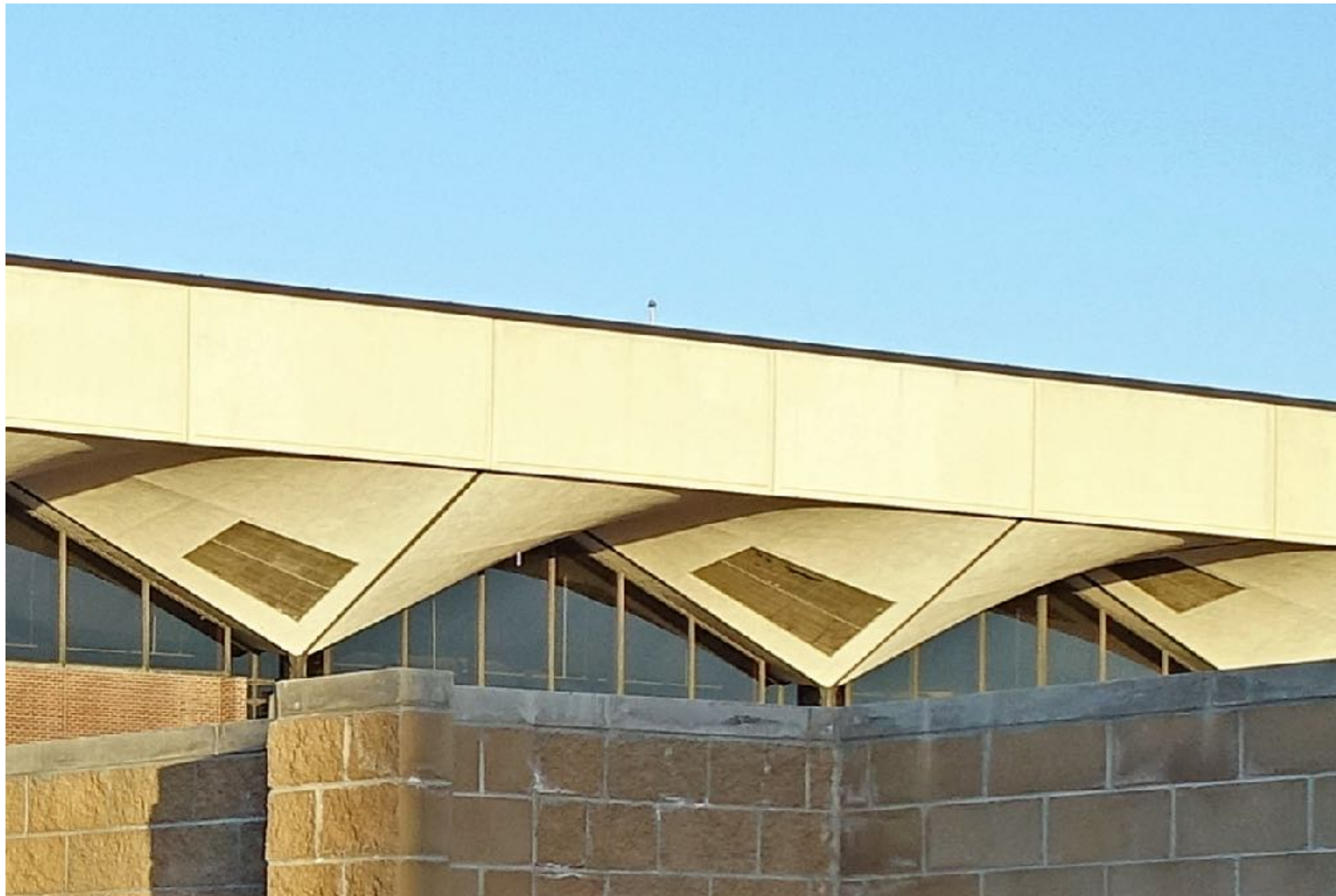
United Airlines Building, Denver
