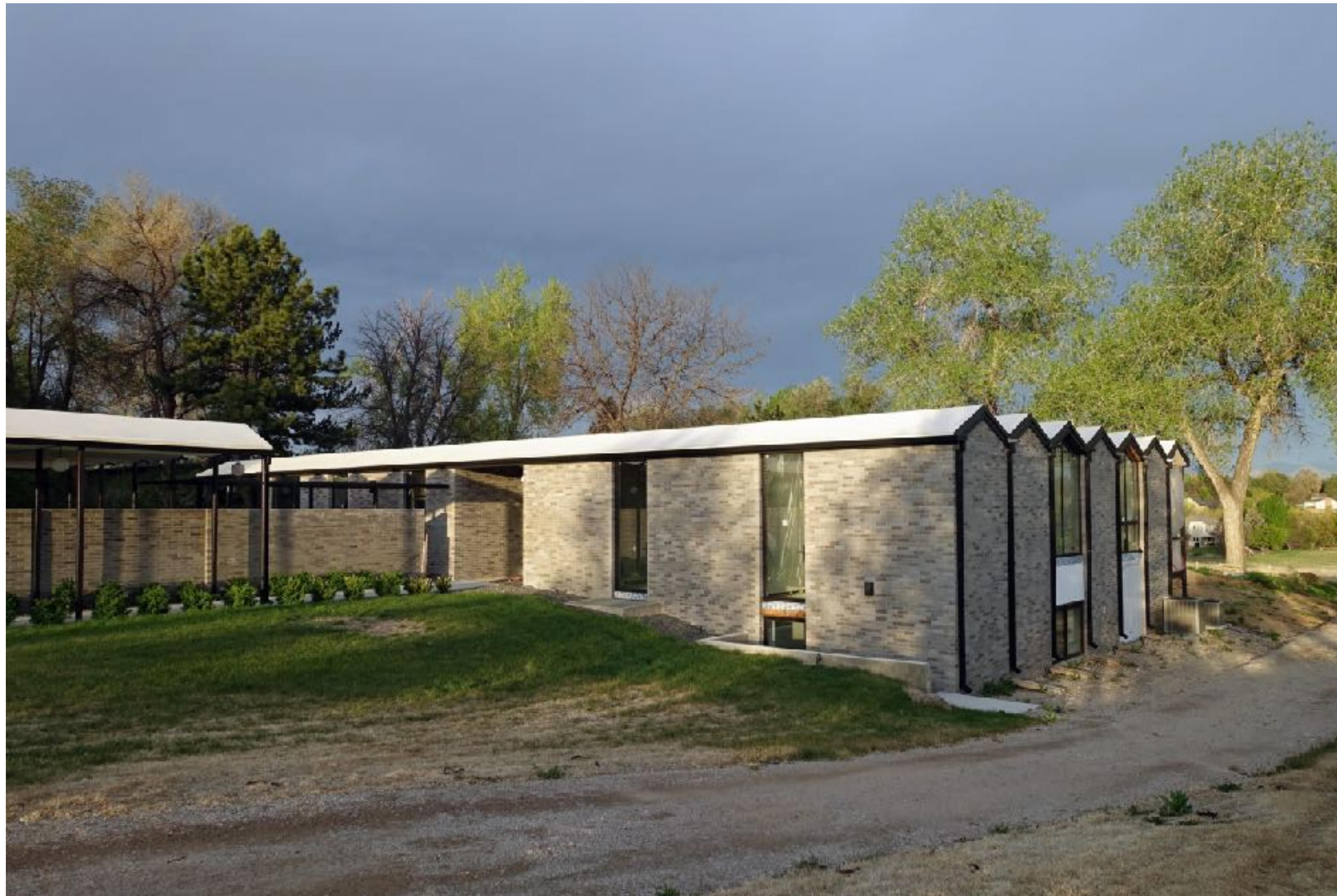
Beck House, Denver
